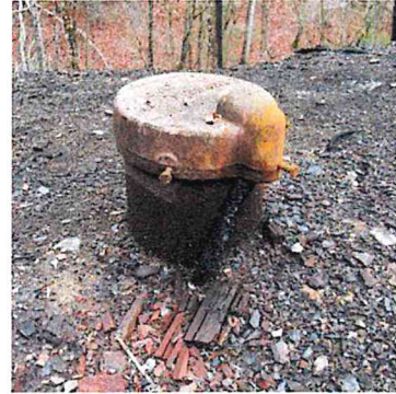
Burned well head after a wildfire. Photo used by permission from the Tennessee Department of Health.
